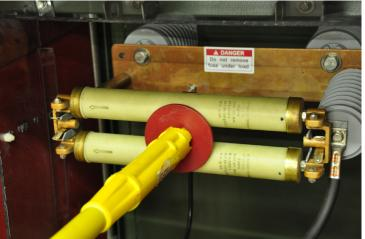
The Elliott Fuse Handling Tool and the operator's insulated shotgun stick have been used to install the parallel fuses in the single fuse mounting.
