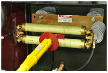
The Elliott Fuse Handling Tool is rotated as shown to remove the Tool.
